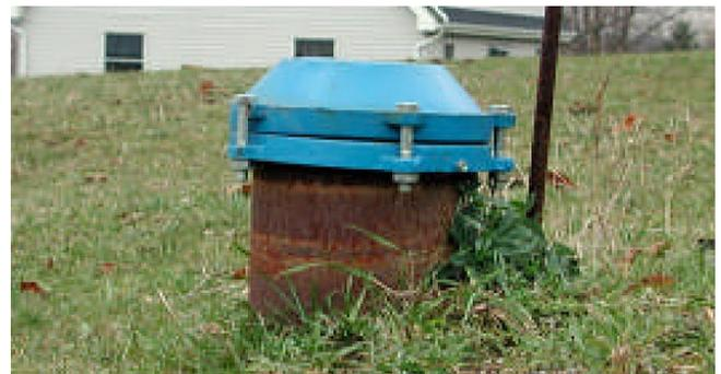
Figure 2. A sanitary well cap installed on a well casing. Note the bolts on the top rather than around the sides of the cap.
