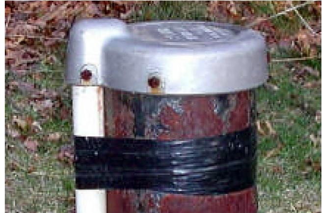
Figure 1. A standard well cap similar to those found on most Pennsylvania wells (note the bolts around the outside of the well cap).
