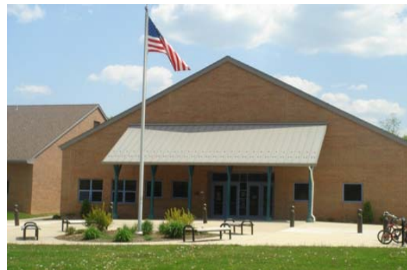
Maple Glen Elementary School
