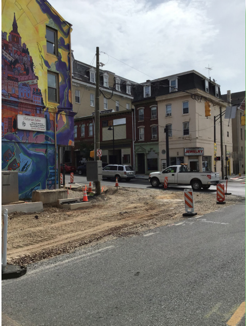
Roadway Construction Dekalb and Lafayette Street
