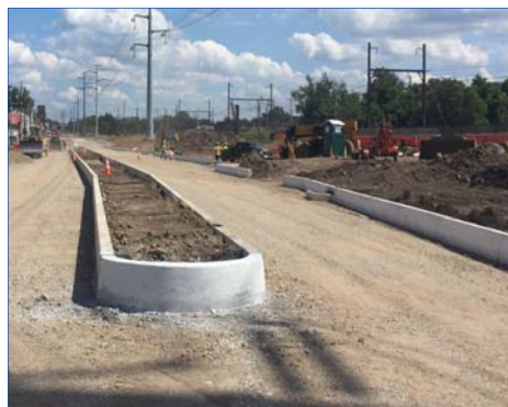
Median and Curb Install East of Dekalb
