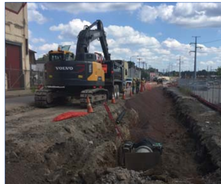
Pipe Installation on Lafayette St. East of Dekalb
