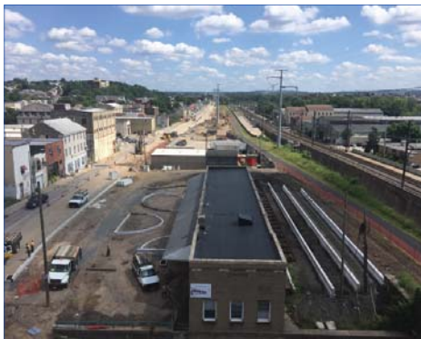
Freight Station with Terrace Walls Installed
