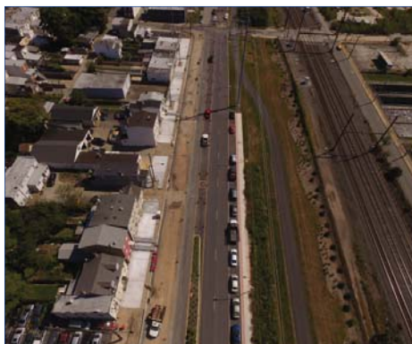
Lafayette Street Sidewalk Construction
