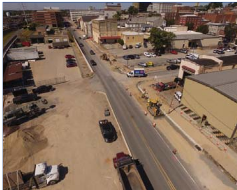
Fine Grade for Roadway Construction
