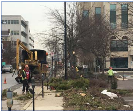
Tree Removal along Lafayette Street
