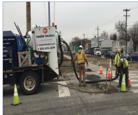
Utility Location Investigation
