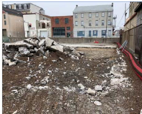
Concrete Demolition at the Frieght Station
