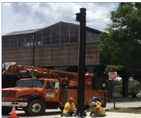
Signal Mast Arm Installation
