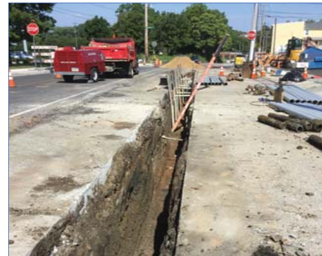
PECO Ductbank Installation
