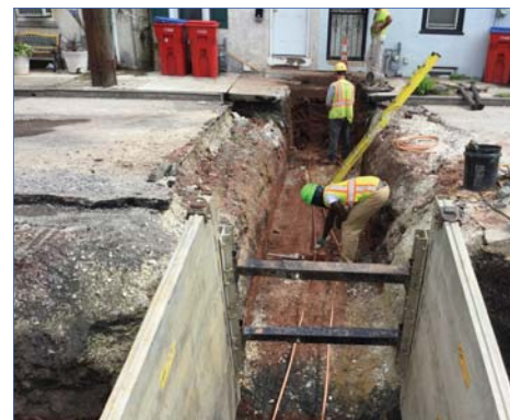
Water Service Installation
