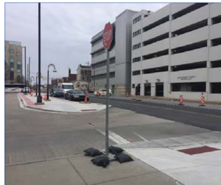
Norristown Transportation Center New Island
