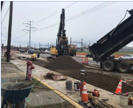
Storm Water Installation
