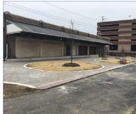
Paver Installation at Freight Station
