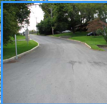
Above - Link between public works yard and high school
