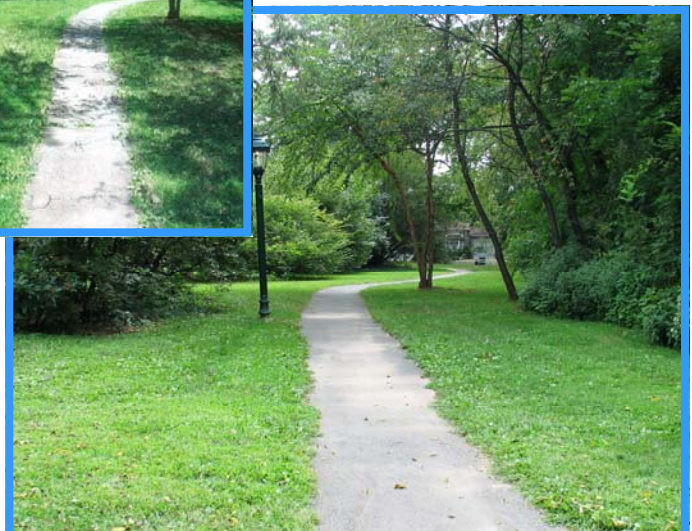
Left and Below - Before and after pathway reconstruction
