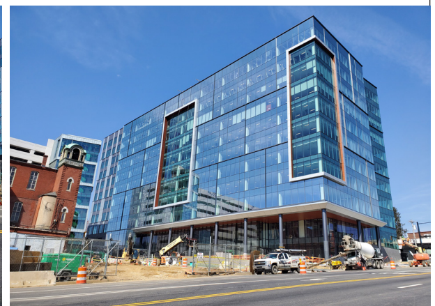
SORA West Office Development
